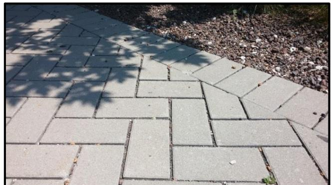
**Permeable pavement at UIC reduces stormwater runoff, meaning less flooding and less demand on the Metropolitan Water Reclamation District**
